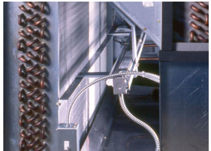
Germicidal Irradiation (UVGI) of 254 nm that constantly irradiates the coil surface.
