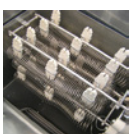
Vertical unit internal factory-installed electric heater
