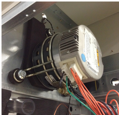
Figure 21: EC Motor
