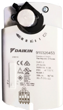
Figure 93: Outdoor Air Damper Actuator
