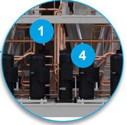
**1 DIRECT EXPANSION HEAT PUMP:** Refrigerant cycle transfers heat from the outdoor air to the indoor space, requiring less electricity to generate heat or cool air.
