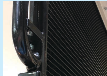
Figure 27: Epoxy Coil Coating
