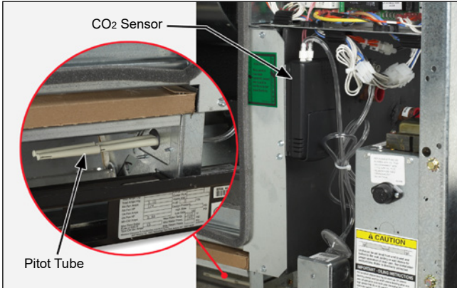
Figure 103: CO 2 Sensor For Demand Control Ventilation
