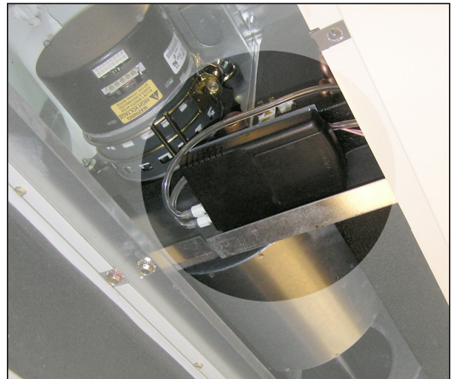
Figure 96: CO 2 Sensor For Demand Control Ventilation
