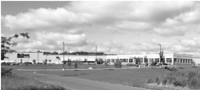
McQuay Air Conditioning plant with over 450,000 square feet of manufacturing space - located in Auburn, New York
