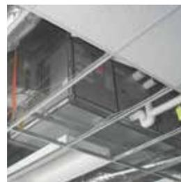
*Suspension rods eliminate need for support brackets*
