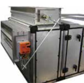
Mixing box section with damper actuator
