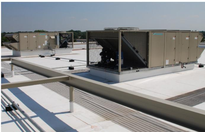
System performance and reliability make Maverick II commercial packaged rooftop systems the ideal solution for new, retrofit or replacement applications on one to three-story buildings. Available in capacities from 15 to 70 tons, they combine the lower installation costs and interior space savings of a roof-mounted system with the operating and maintenance efficiencies of central heating and cooling systems.
