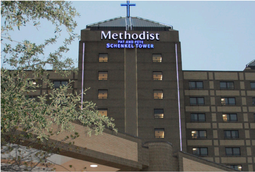
Methodist Dallas Medical Center achieved an 18-month payback on a new HVAC system that includes a 2,000-ton Daikin dual-compressor centrifugal chiller.
