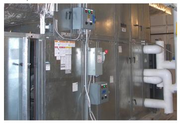
One of three large Daikin Vision air handling units installed for the vehicle service are
