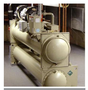
The two compressors of the Magnitude chiller operate on a common refrigerant circuit, improving system reliability.
