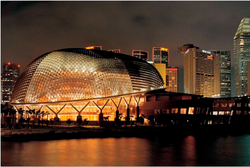
The multi-activity performing arts facility's main architectural feature consists of two huge, domed Mero latticed supporting structures that comprise the roof.
