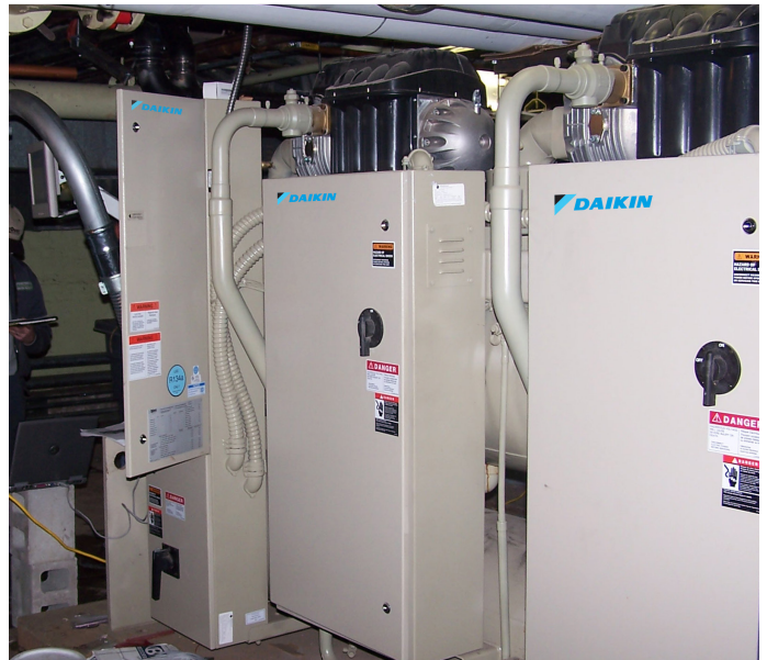
The Magnitude chiller was installed next to an older screw compressor chiller and the new chiller is dramatically quieter than the other machine.
