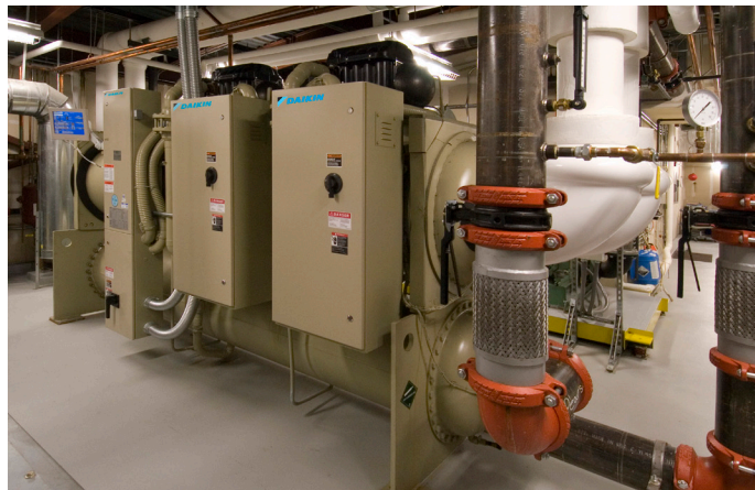
The 300-ton Daikin Magnitude chiller was selected for the Alumni Center based on its compact footprint, part-load performance, and quiet operation.
