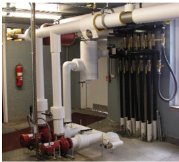
A series of 35 holes, six inches in diameter were bored 400 feet below the parking lot behind City Hall and connected to a valve manifold in the basement of the building. From there, small pipes carry the heated or cooled water to the individual heat pumps throughout Auburn City Hall.
