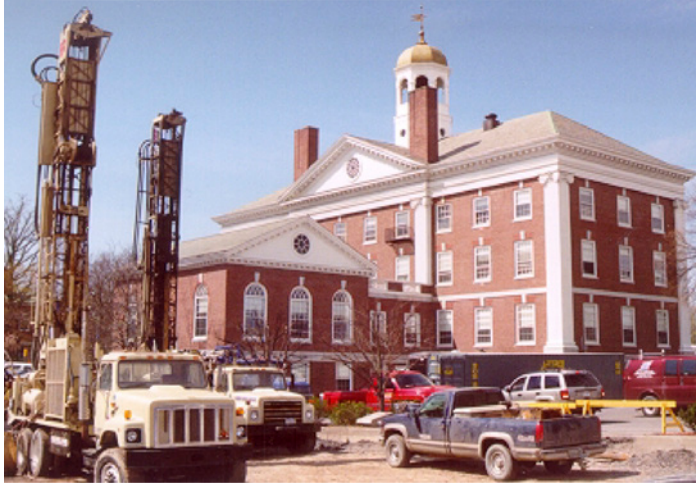
A series of 35 holes, six inches in diameter were bored 400 feet below the parking lot behind City Hall and connected to a valve manifold in the basement of the building. From there, small pipes carry the heated or cooled water to the individual heat pumps throughout Auburn City Hall.
