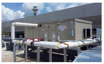
44 new (in addition to 76 existing) Daikin Skyline outdoor air handlers provide air handling requirements for the airport's terminals.
