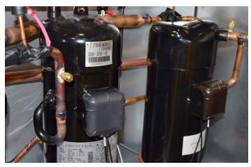
Rebel's modulating inverter scroll compressor allows for superior comfort control, energy efficiency, and cost savings than typical compressors.
