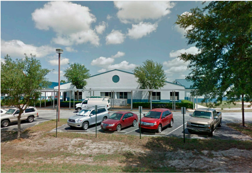
West Hernando Middle School felt effects of outdated HVAC technology chose Daikin for DOAS and VRV solutions that deliver comfort for occupants and a quick ROI for the school district.
