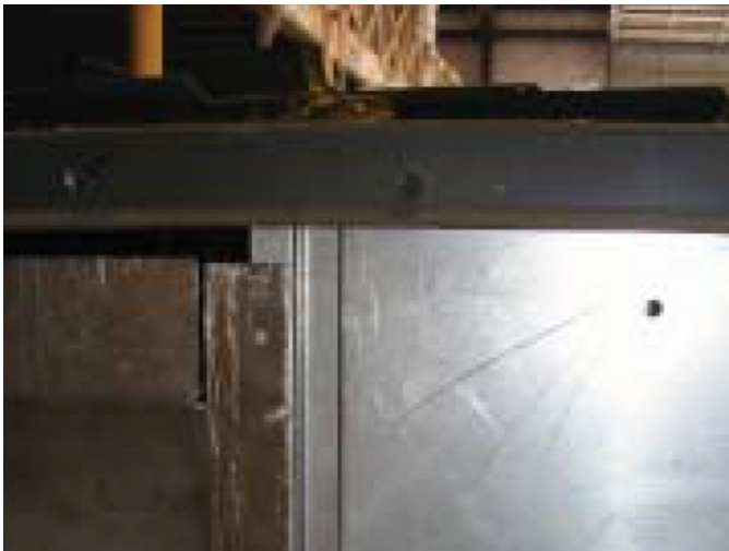
Figure 25: Attached Mixed Air Sensor on Blower
