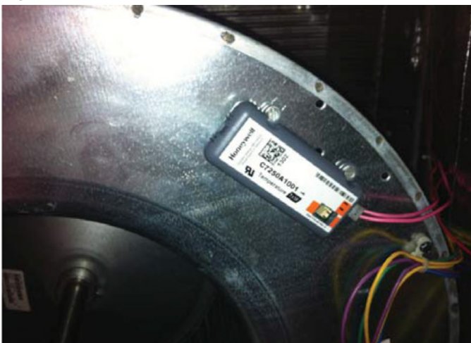
Figure 25: Attached Mixed Air Sensor on Blower
