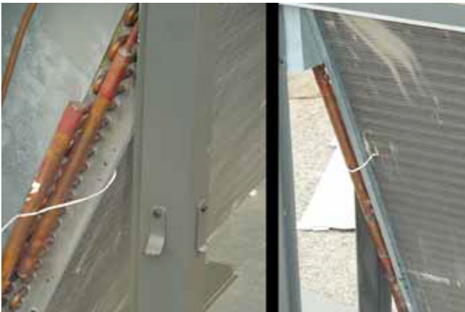
Figure 82: Mounting Temperature Probe near Liquid Line Tube
