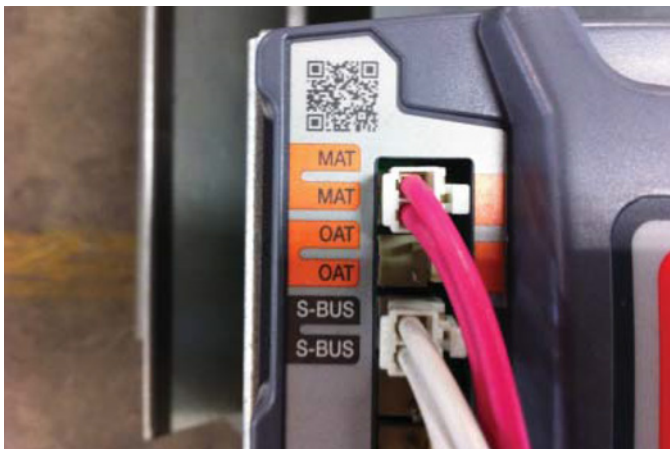
Figure 1: Mixed Air Sensor Connections
