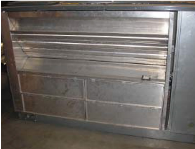
Figure 24: Correct Damper Positioning—Detail
