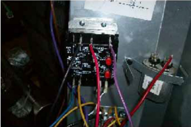
Figure 81: Mounting Temperature Probe near Condenser Coil
