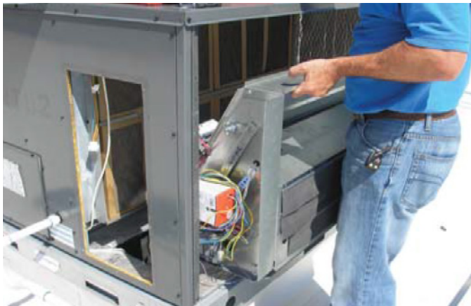
Figure 7: Installing the Internal Damper Rack
