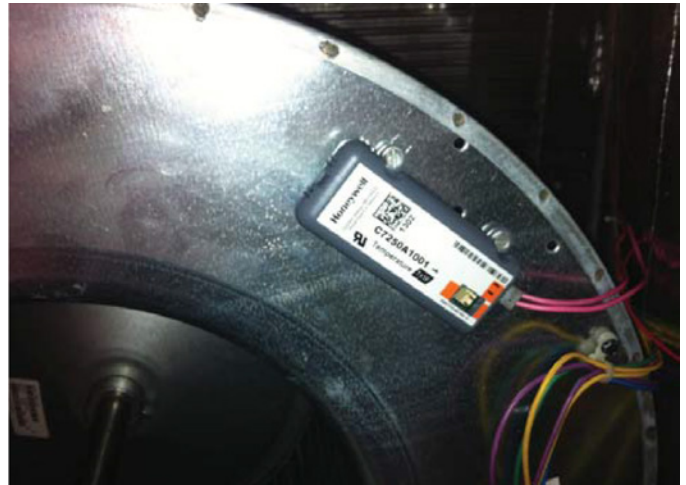
Figure 9: Attached Mixed Air Sensor on Blower
