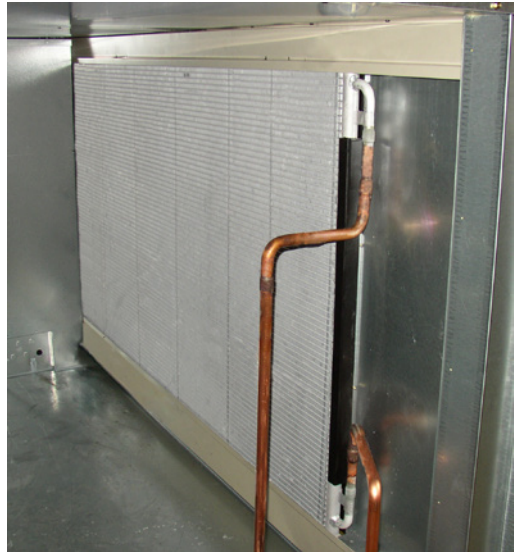
Figure 2: Typical Modulating Hot Gas Reheat Coil
