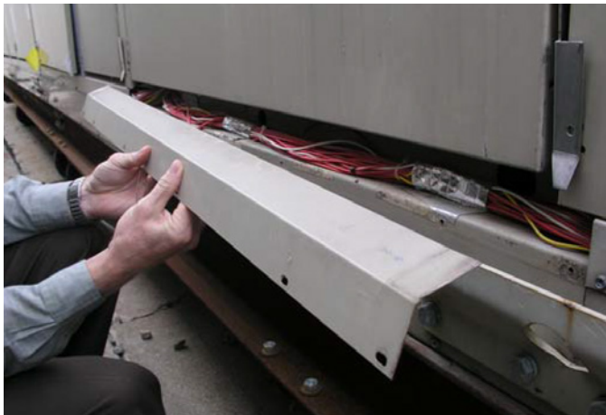
Figure 2: Control Wiring Raceway
