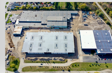
Left: Precast In-Progress Right Upper: Precast Complete Right Lower: Site Plan Aerial View
