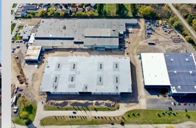
Left: Precast In-Progress Right Upper: Precast Complete Right Lower: Site Plan Aerial View
