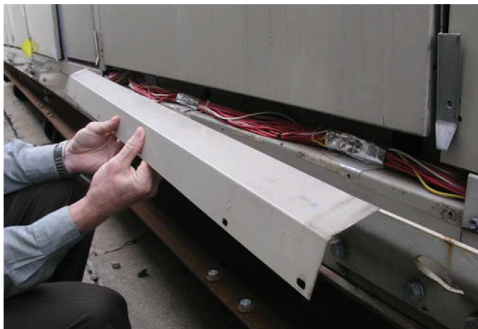
Figure 2: Control Wiring Raceway
