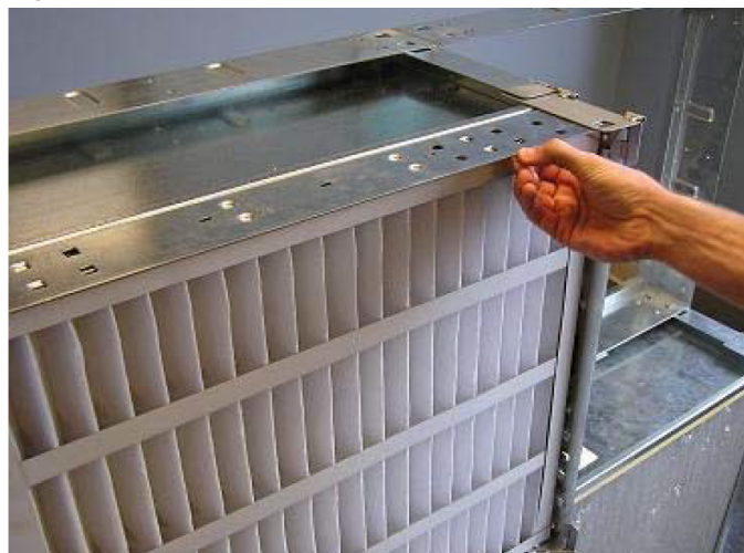
Figure 115: Installation of Prefilter Into Frame
