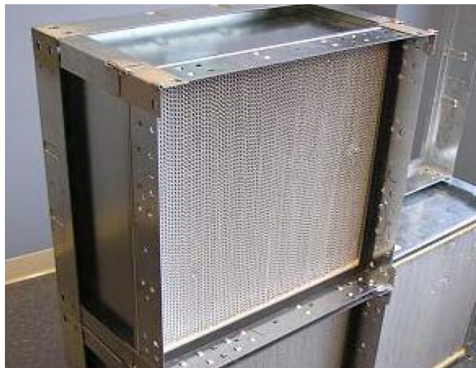
Figure 114: Properly Installed HEPA Filter
