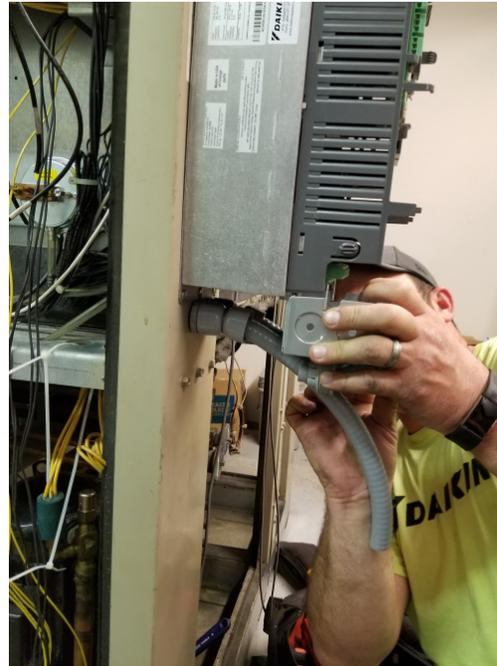
**Figure 12: VFD Installation**
