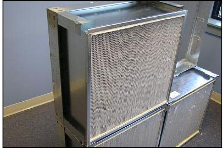
Figure 124: Filter Placed Inside of Frame
