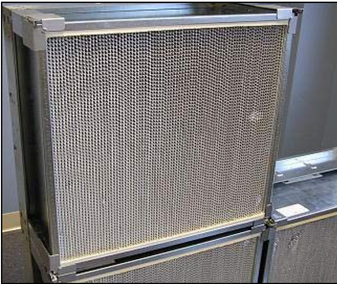
Figure 128: Properly Installed Filter Inside of the Frame
