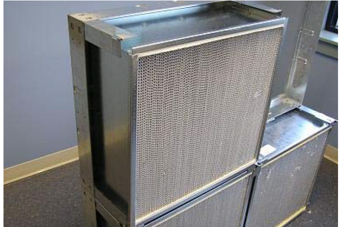
Figure 111: Filter Placed Inside of Frame
