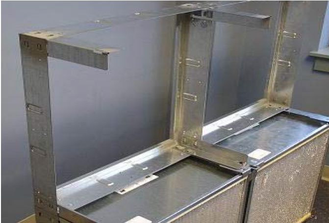
Figure 109: Frame with Leg Extensions Installed
