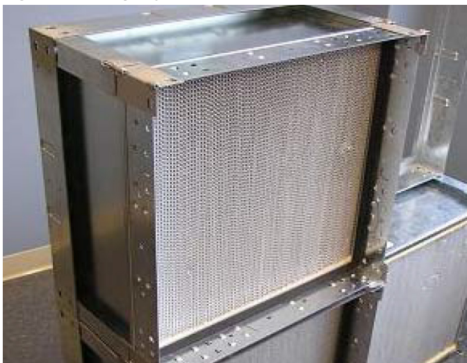
Figure 120: Properly Installed HEPA Filter
