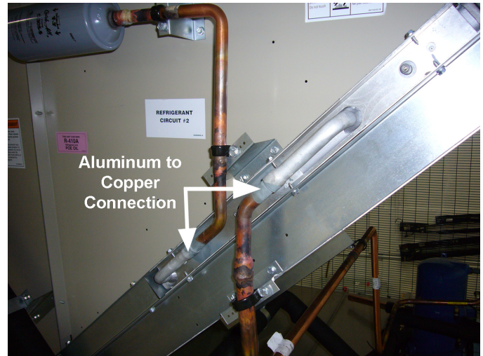
Figure 66: Aluminum/Copper Connection
