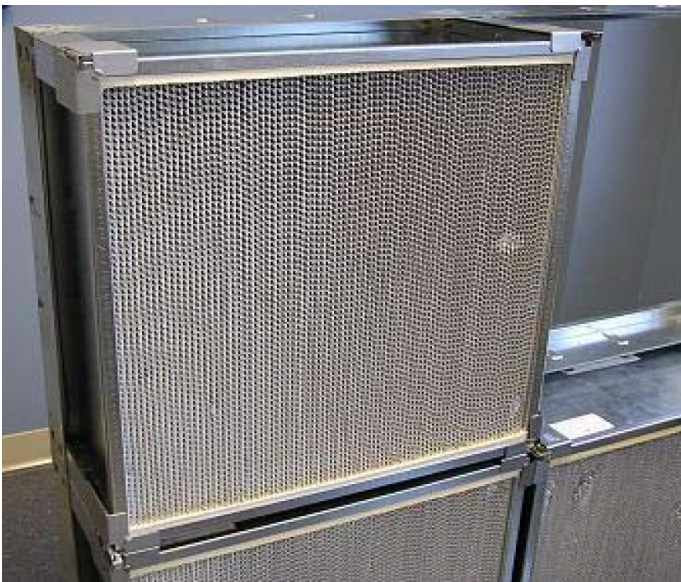
Figure 49: Properly Installed Filter Inside of the Frame
