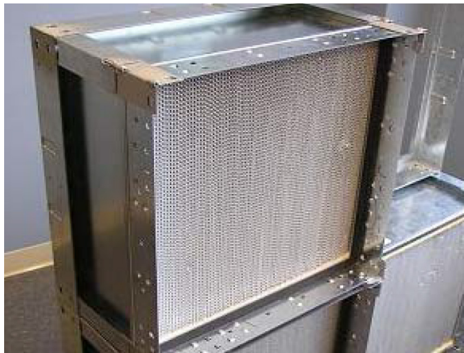
Figure 54: Properly Installed HEPA Filter
