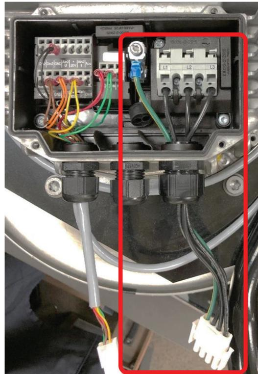
**Figure 69: Single Fan Control Panel - High Voltage Wiring (in red); Low Voltage Wiring (in blue)**
