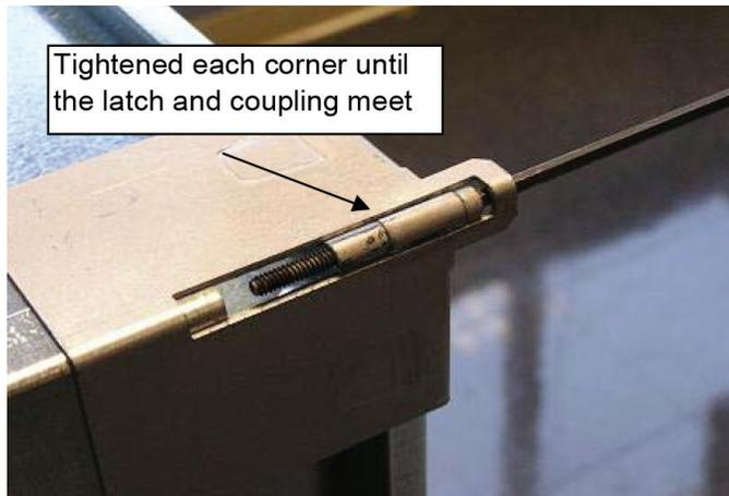
**Figure 27: Properly Installed Filter Inside of the Frame**
