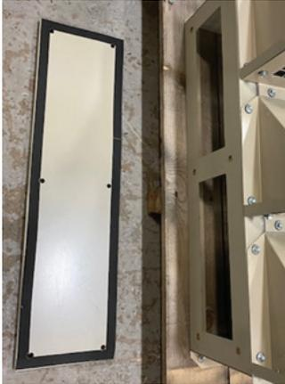
**Figure 90: Side flange to be secured once side panel is removed**
