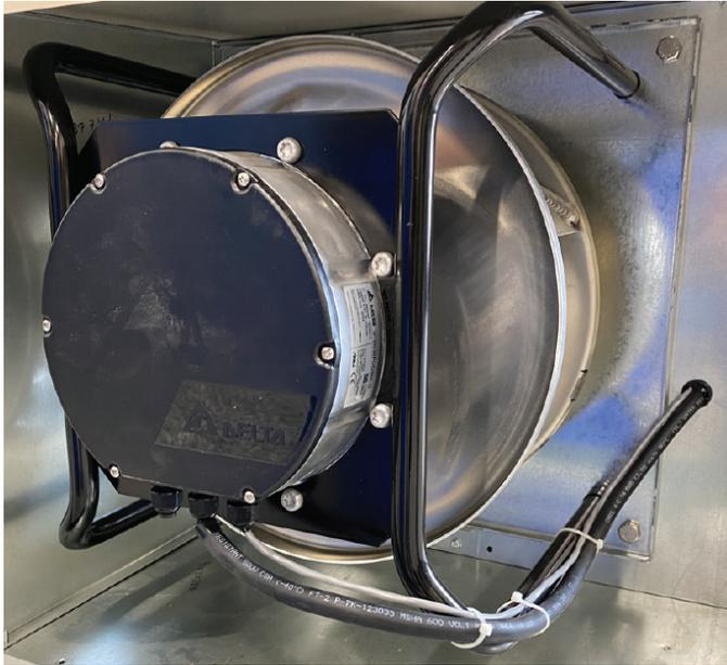
Figure 81: Delta Motor - Control Wiring with No Controls
