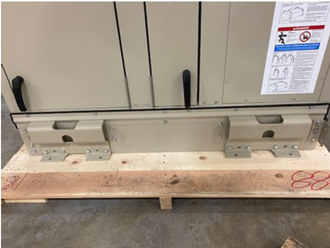
Figure 100: Lifting lugs located on base rail
