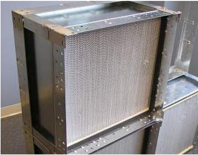
Figure 35: Properly Installed HEPA Filter
