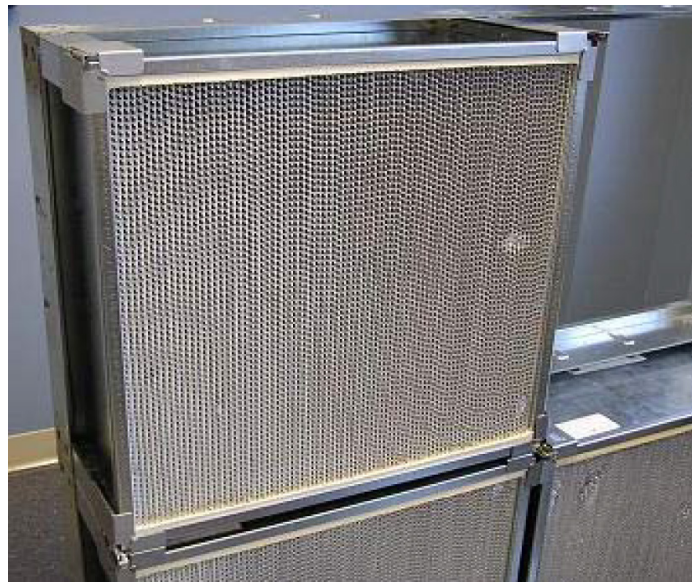
Figure 29: Properly Installed Filter Inside of the Frame
