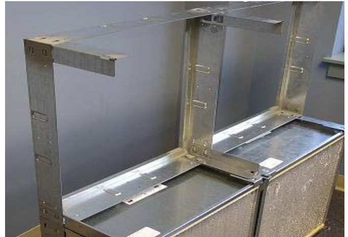
Figure 23: Insert HEPA Filter into Frame, until the Gasket Comes in Contact with the Holding Frame
