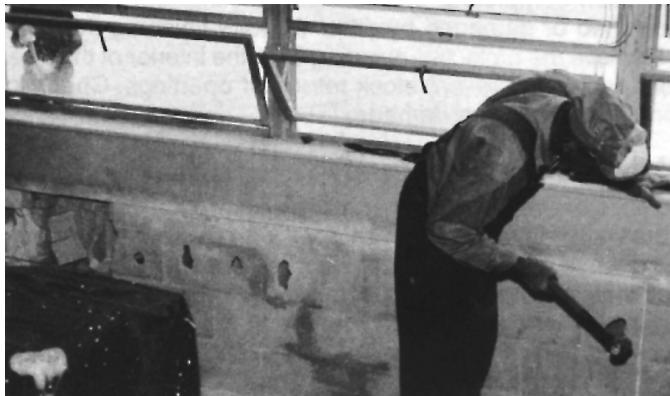
Figure 13: The interior wall is knocked out in the area cut for the wall sleeve
