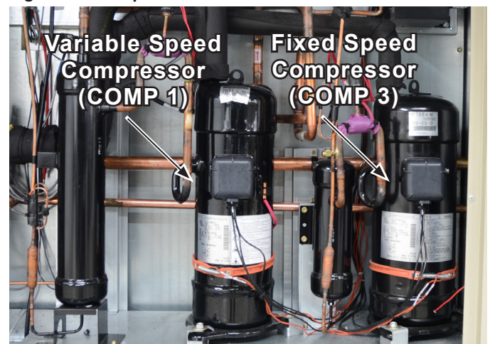
Figure 21: Compressor Tandem on Medium Cabinet
