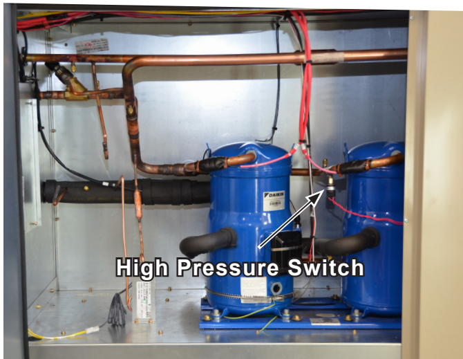
Figure 34: High Pressure Switch
