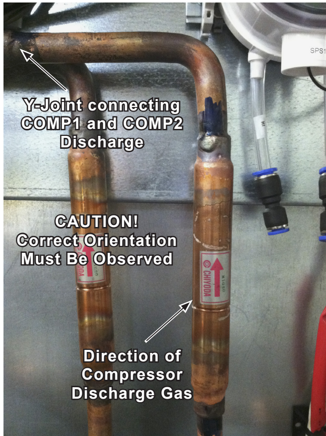
Figure 25: Discharge Line Check Valves on Large Cabinet (7.5T) Heat Pump (DPH)
