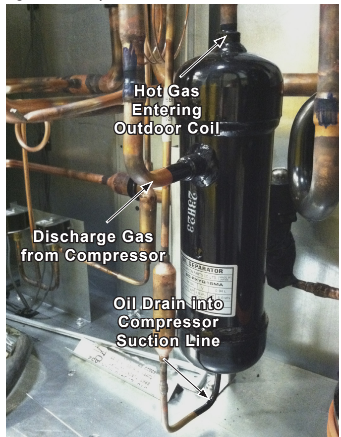
Figure 23: Oil Separator
