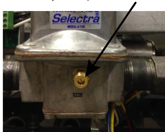
Figure 56: Pressure Adjustment Screw (shown with blue cap removed)
