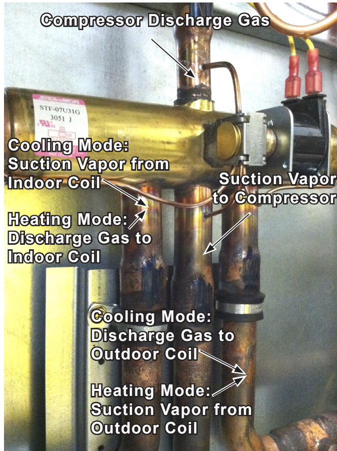
Figure 28: Four-Way Valve
