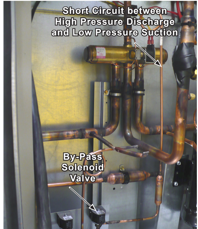
Figure 29: By-pass Solenoid Valve
