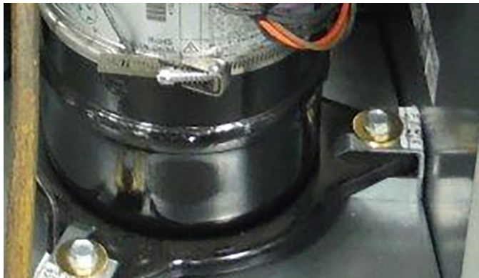
Figure 19: Compressor Brackets
