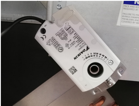
Figure 12: Face & Bypass Actuator
