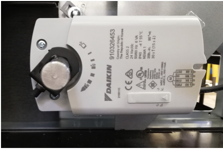
Figure 11: Outdoor Air Damper Actuator
