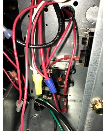
16. Connect (Orange) wires 25A, 26A and 27A from the kit, to the proper terminal pins on the relays.
