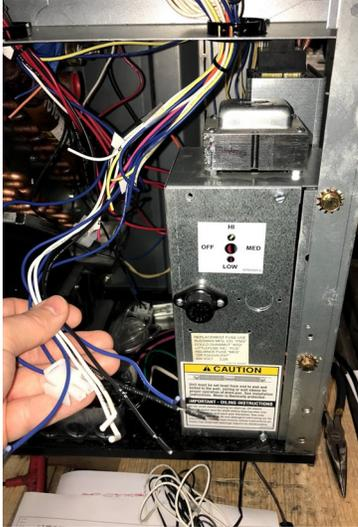
27. Remove the existing floating-point OA damper actuator.
