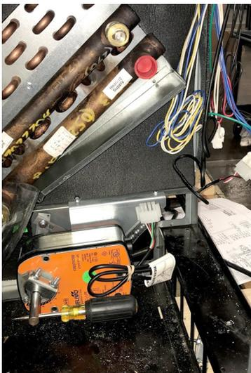
29. Connect the Molex with the new jumper conversion harness provided with the retrofit kit.
