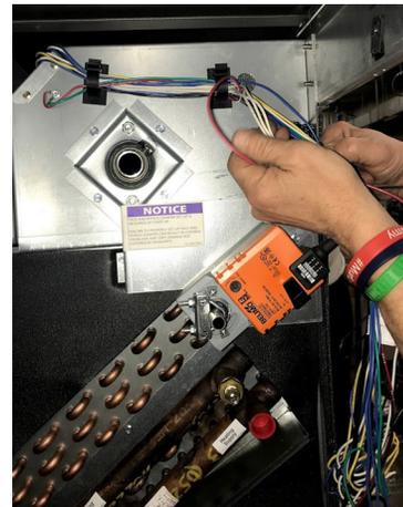
33. Route all wires from the damper actuators to the control box and in through the left grommet opening.
