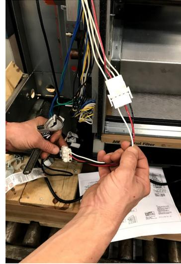
30. Disconnect the F&BP damper actuator on units equipped with F&BP dampers.
