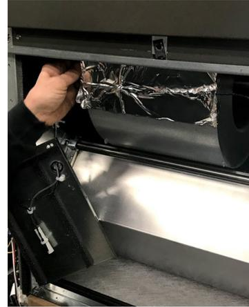
**Note:** *The 10K DAT sensor provided with the kit is pre-wired but the existing DAT wire can be reused.*
