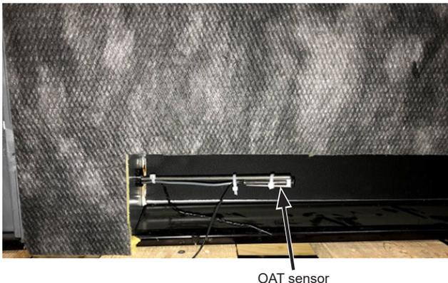
43. Remove the outside air temperature sensor and replace it with the OAT included with the retrofit kit.
