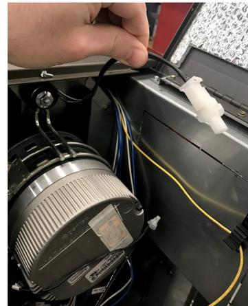
38. Plug the 10K thermistor connector to terminal H9 (pins 1 & 2) on the MicroTech control board. Refer to Figure 36 on page 11
