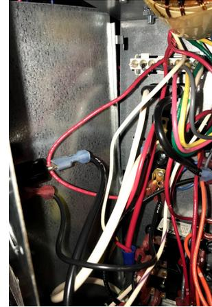
**Figure 20: Transformer Control Box with Wiring from SW1**
