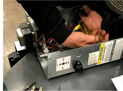
**Figure 9: Relays Installed in Transformer Control Box**
