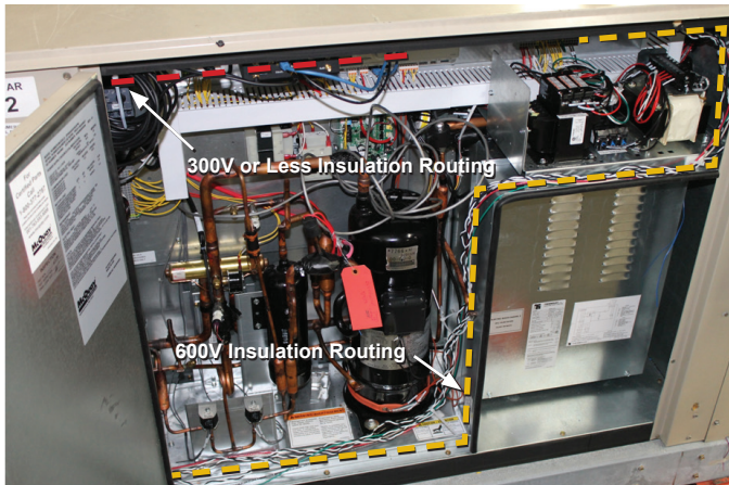
Figure 74: Typical Rebel Wire Routing
