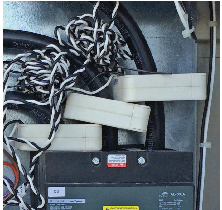
Figure 43: CT Installation
