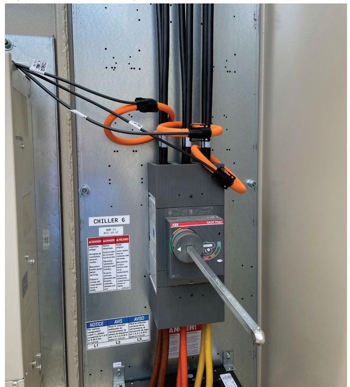
Figure 36: Installed Rogowski Coils
