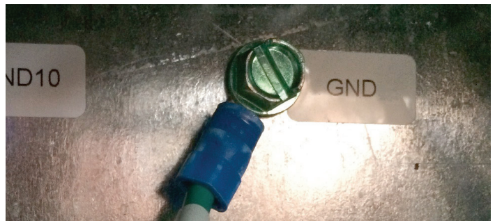
Figure 47: Typical Grounding Lug
