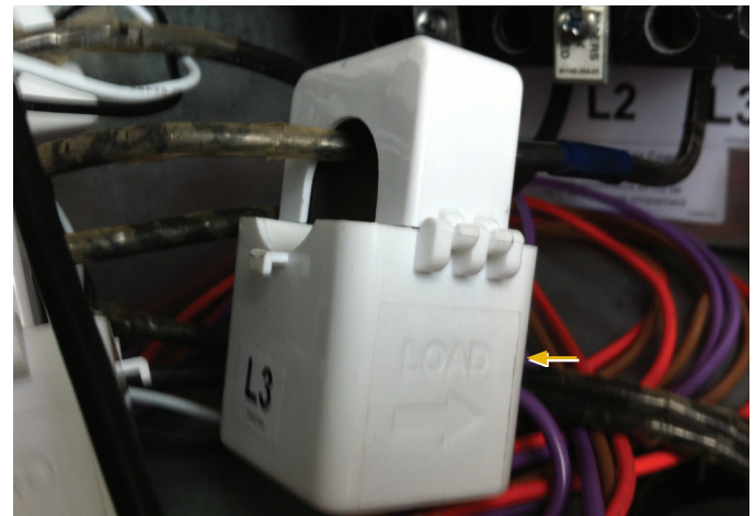
Figure 91: CT Installation
