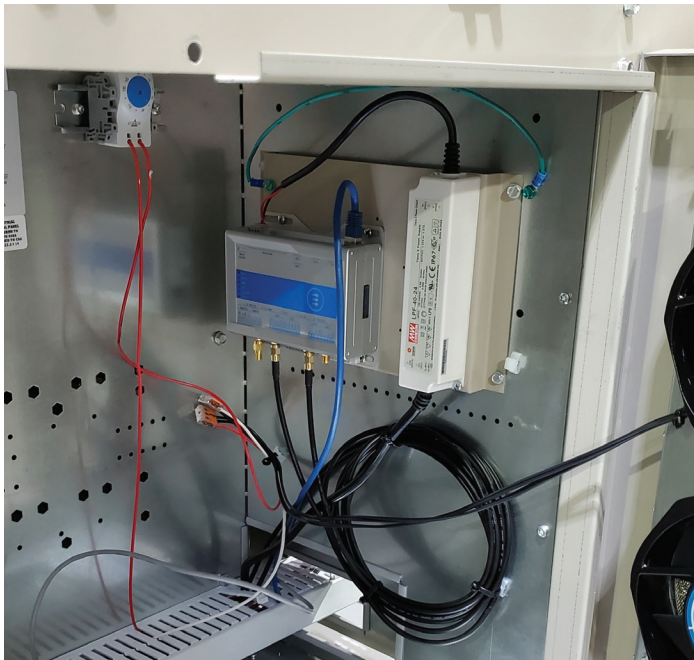
Figure 71: DPSA (Rebel Applied) Gateway Bracket Mounting Location
