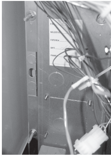
Figure 79: Slide the Unit Up to the Wall Sleeve Threaded Studs
