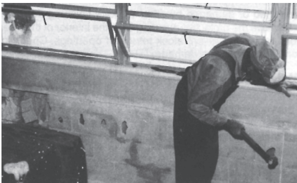
Figure 13: The Interior Wall is Knocked out in the Area Cut for the Wall Sleeve
