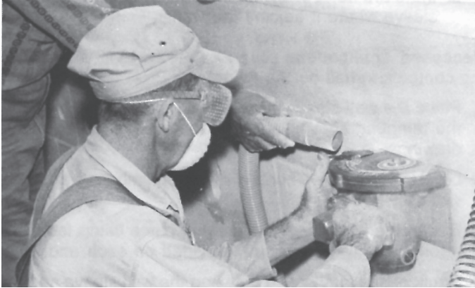
Figure 12: The Interior Wall Opening is Cut
