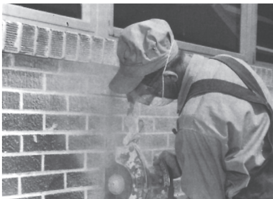
Figure 10: Cutting the Outside Wall Rough Opening Slightly Larger Than the Size of the Louver
