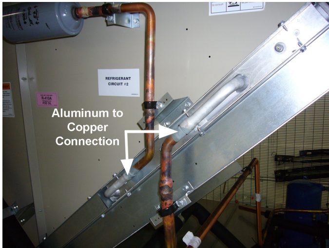
Figure 59: Aluminum/Copper Connection
