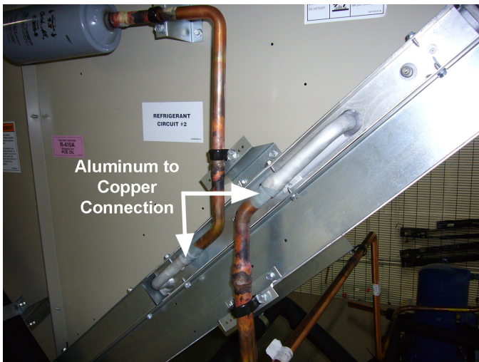
Figure 78: Aluminum/Copper Connection
