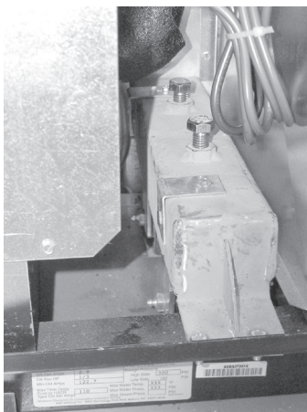
Figure 74: (Optional) Indoor Section Caster Shown in Right End Compressor Compartment
