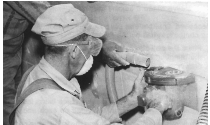
Figure 12: The Interior Wall Opening is Cut
