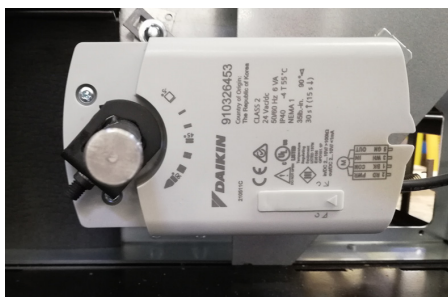
Figure 117: Outdoor Air Damper Actuator
