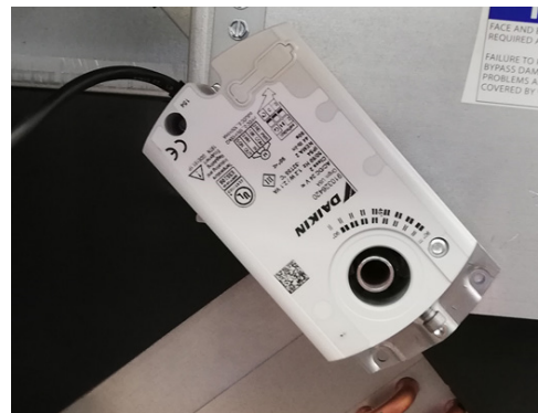
Figure 118: Face & Bypass Actuator
