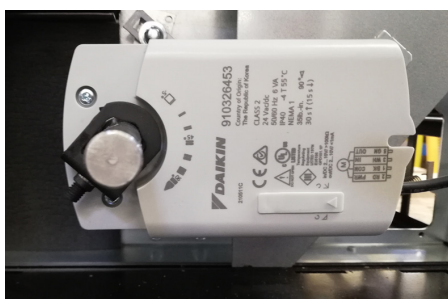
Figure 117: Outdoor Air Damper Actuator
