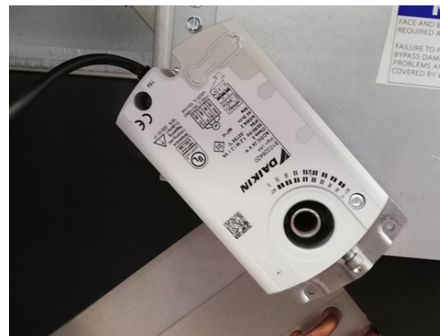
Figure 118: Face & Bypass Actuator
