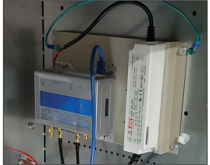
Figure 11: Generation 2 Gateway Installed on Control Panel Backplane
