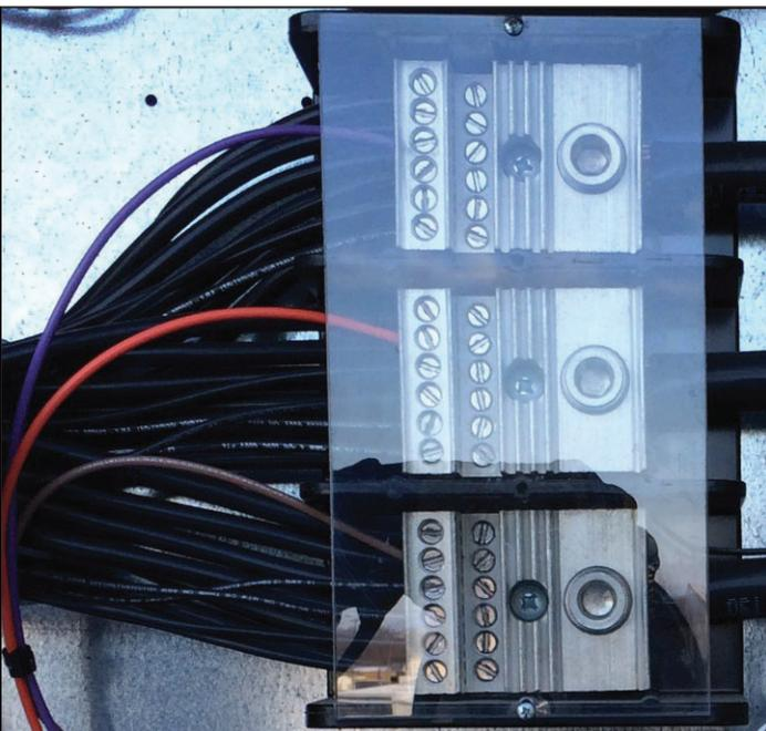
**Figure 18: EMM Connection to Fuse Block**
