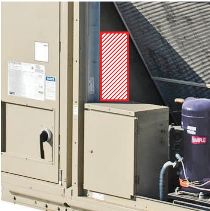
Figure 52: Recommended Location for RoofPak Control Enclosure Penetration
