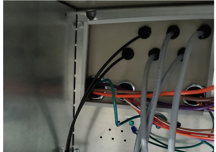
Figure 53: Rebel Applied Cabinet Knockouts
